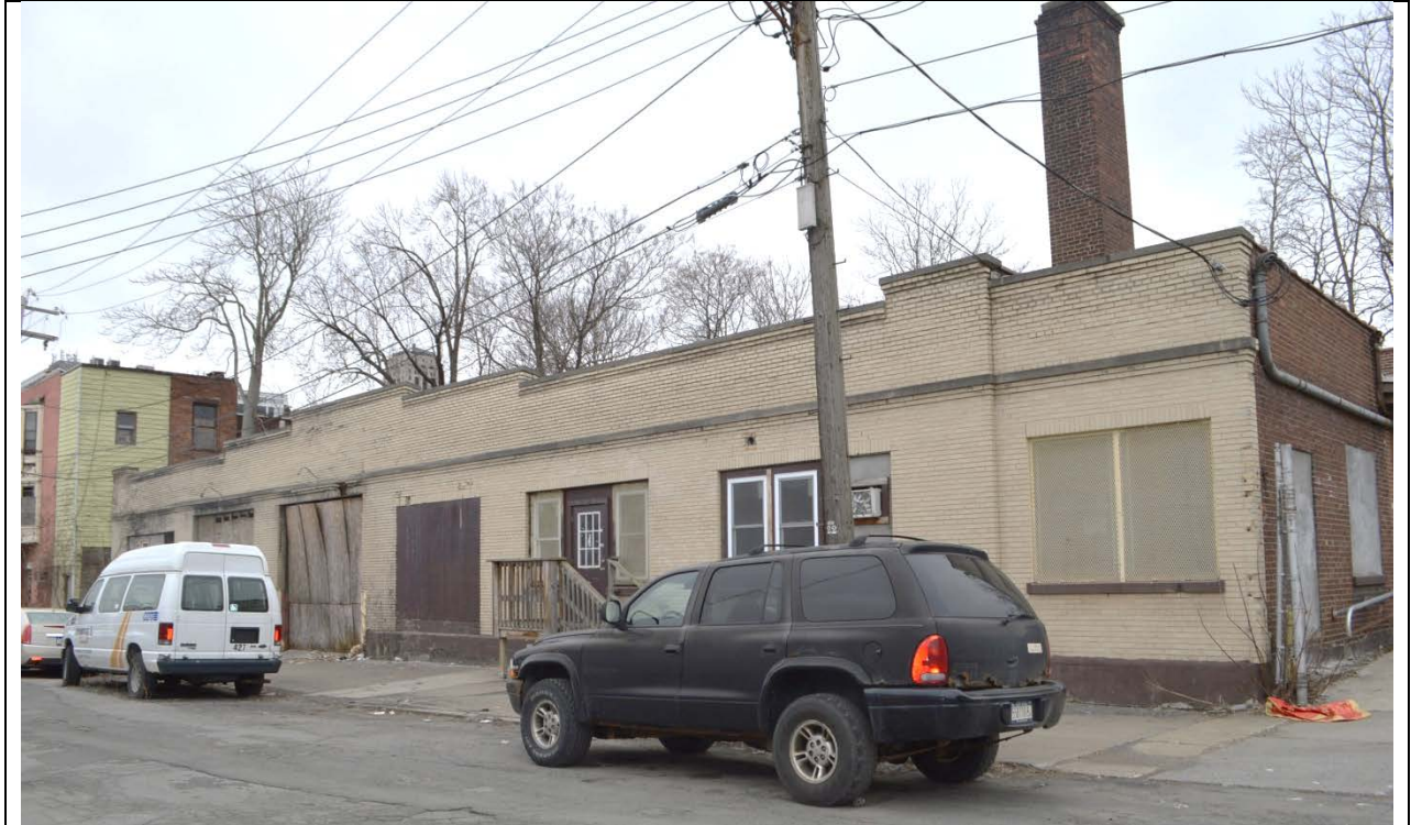
228-232 Spruce Street (Presently referred to as 222 Spruce St.) – front (north) elevation
