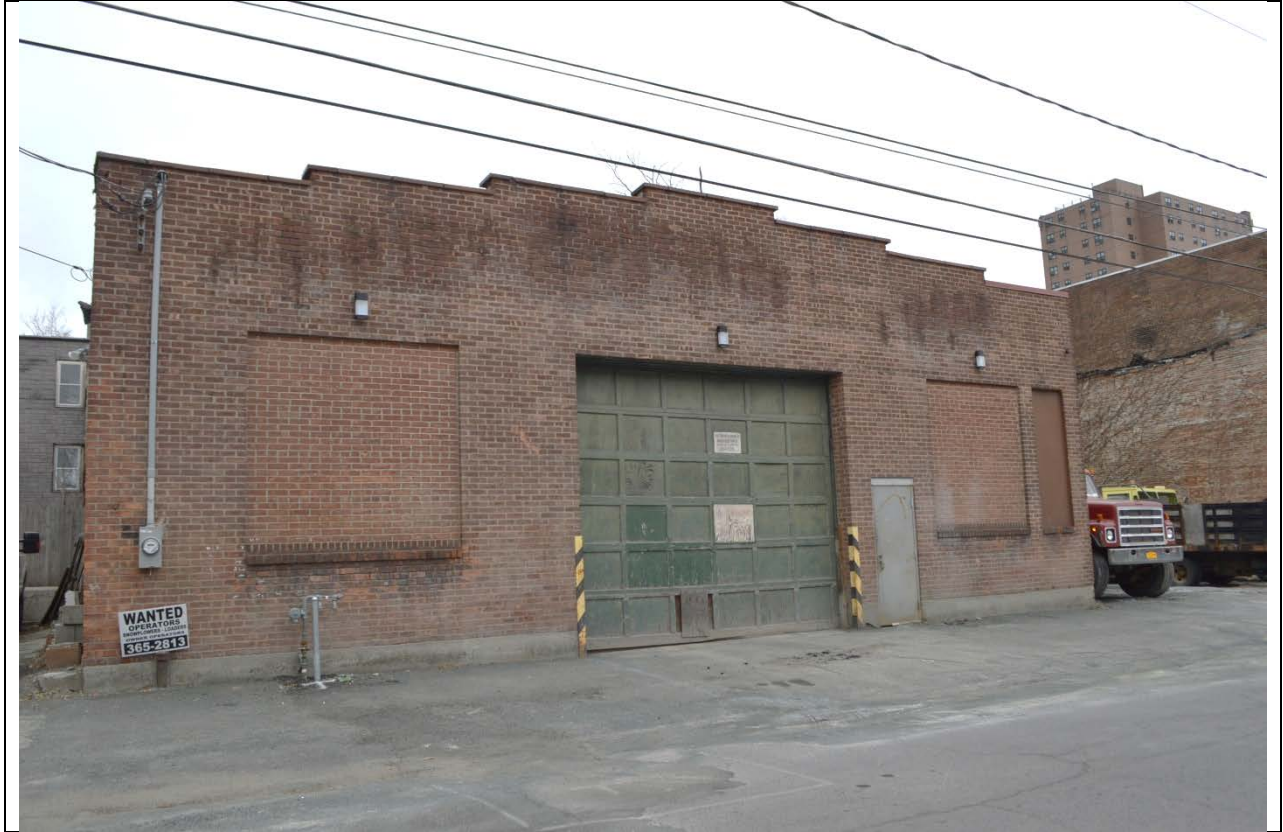
196 Elk Street - front (north) elevation
