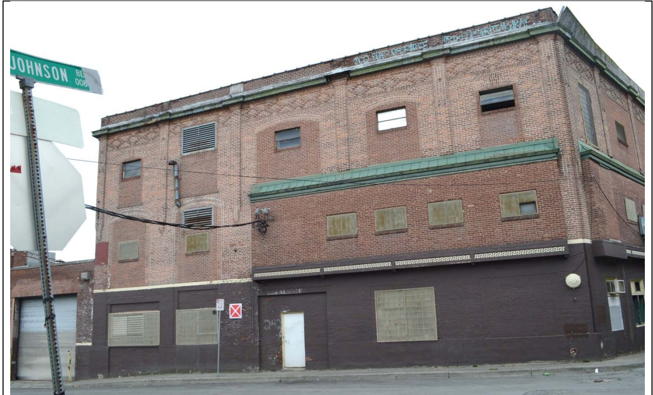
64 Henry Johnson Boulevard (Presently referred to as 242 Spruce St.) – view of Spruce Street elevation.
