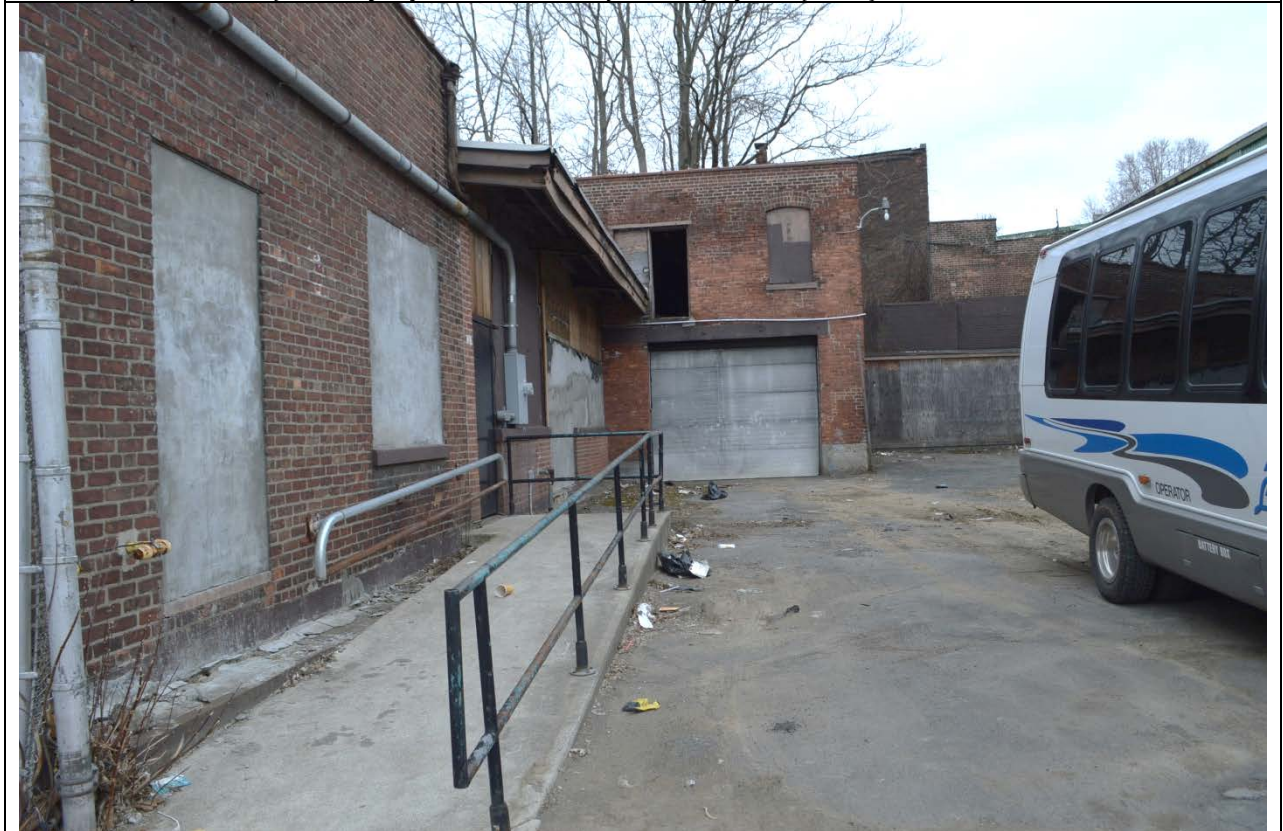
228-232 Spruce Street (Presently referred to as 222 Spruce St.) – side (west) elevation
