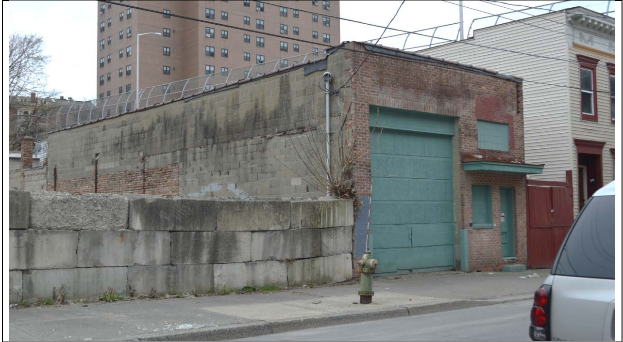
228 Elk Street – view of side (east) and front (north) elevations
