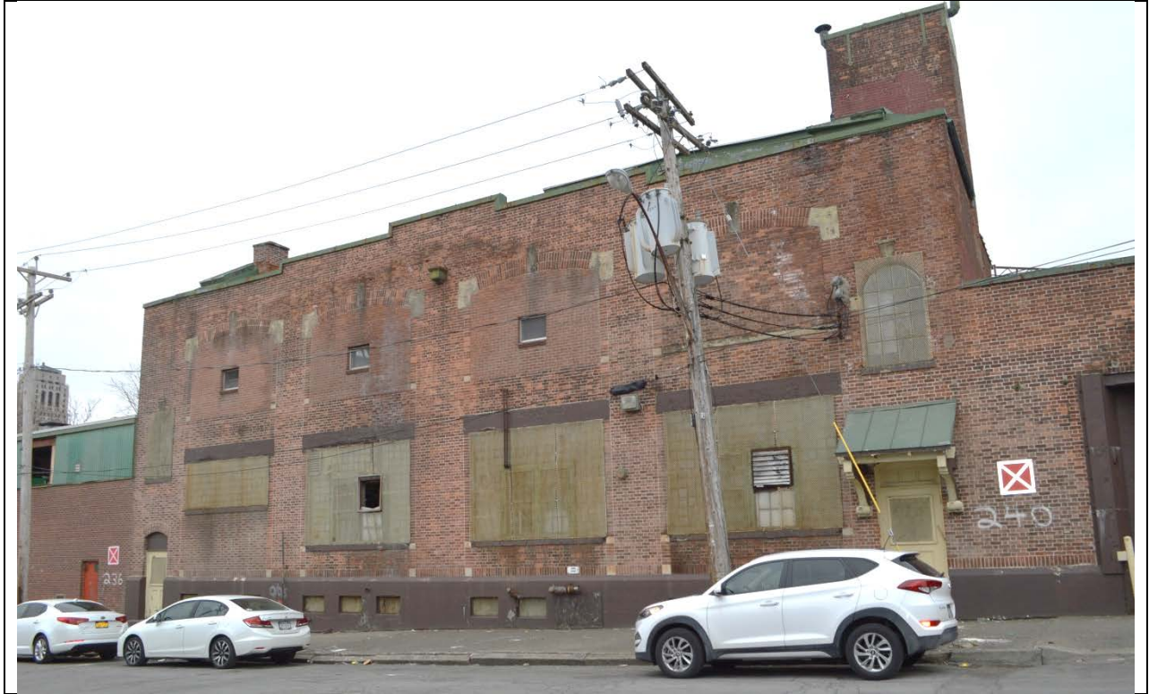
242 Spruce Street (Presently referred to as 240 Spruce St.) – front (north) elevation
