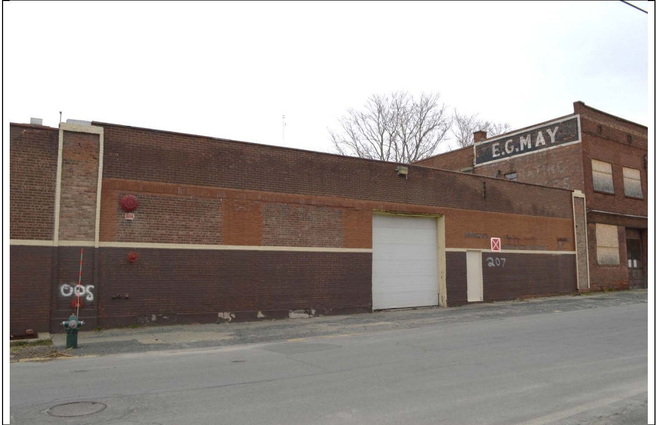
201 Elk Street (Presently referred to as 207 Elk St.) – view of front (south) elevation.
