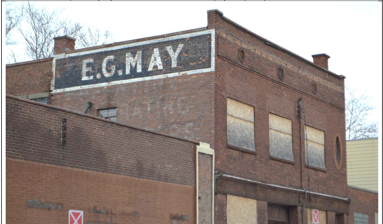
199-201 Elk Street (Presently referred to as 201 and 197 Elk St.) – view of painted wall sign on west elevation.
