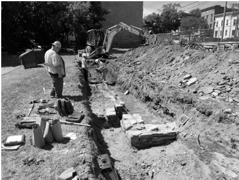
Photo 5. West end of Trench 4 with exposed wall foundations. View northwest.
