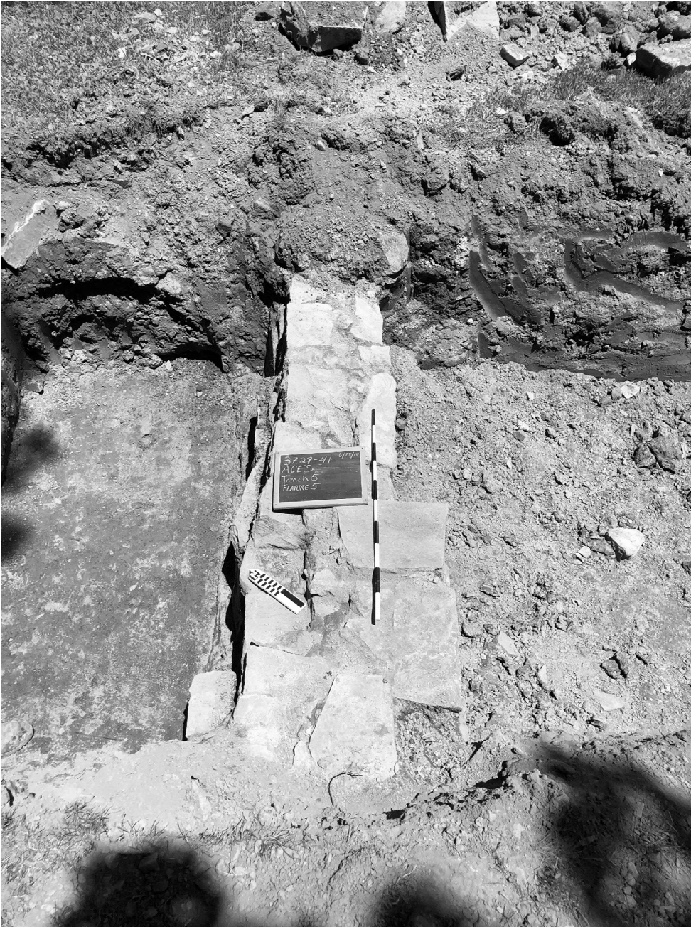
Photo 24. Foundation wall from Trench 5 with reddish brickyard deposit to the left in the foreground. View northeast.
