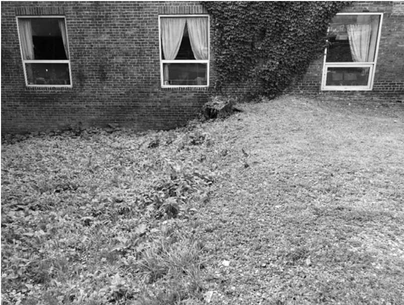
Photo 3. Difference in elevation and slope between the APE (right) and neighboring property (left) reflecting demolition and grading in the APE. View southwest.
