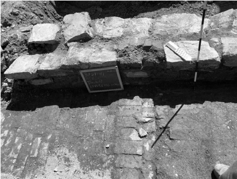
Photo 18. Brick dividing wall inside of 238 Clinton Avenue. Note that it was built into a niche in the cut stone foundation and that the direction of bricks in the floor on either side changes from north/south to east/west. View southwest.
