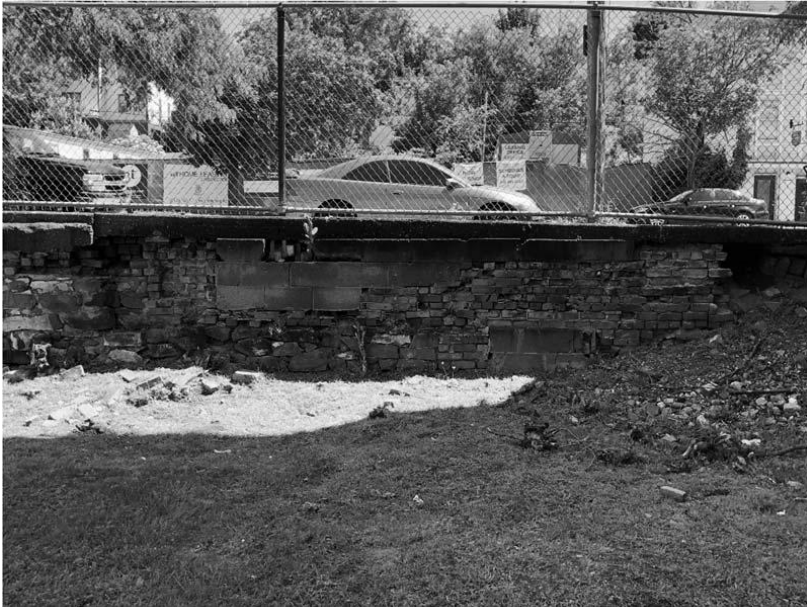
Photo 1. Retaining wall between the APE and Clinton Avenue consisting of remains of the front foundations of now demolished structures under investigation. View northeast.
