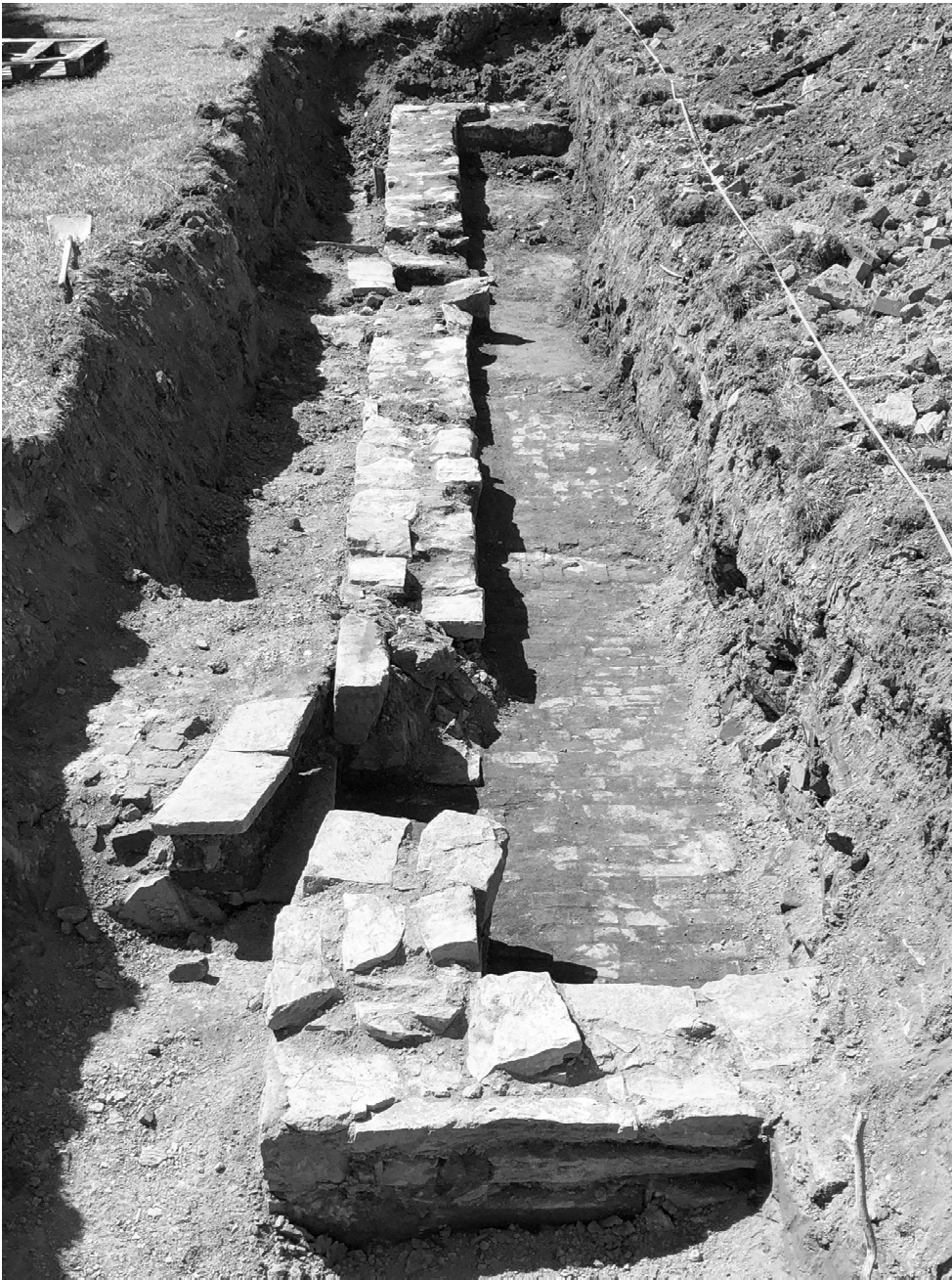
Photo 12. Wall foundations and floors of structures at 238 and 240 Clinton Avenue. View northwest.
