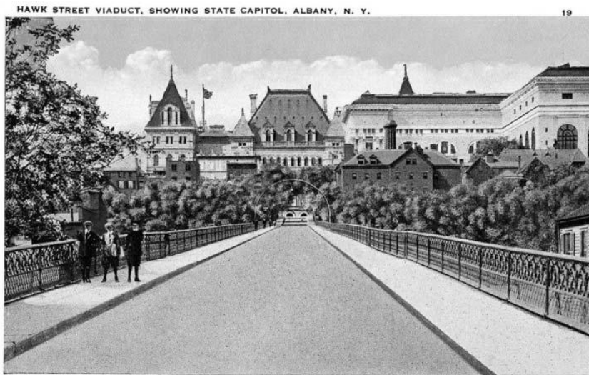
Figure 6. Postcard showing the Hawk Street Viaduct (1890-1970) circa 1900. https://friendsofalbanyhistory.wordpress.com/2018/01/23/the-hawk-street-viaduct/
