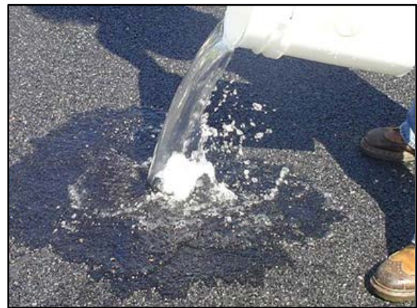
Figure 12. Pervious Pavement Test by Pouring Water Source: Philadelphia Water Dept.
