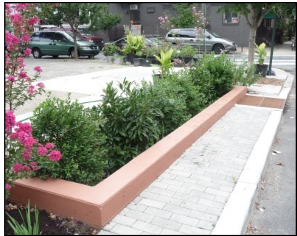
Figure 8. Curbside Stormwater Planter Source: Philadelphia Water Department
