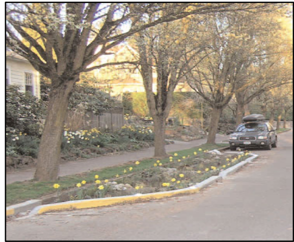
Figure 7. Philadelphia Water Dept. - Curb Extension
