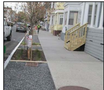
Figure 23. GI Project located at Intersection of Quail Street and Elberon Place.
