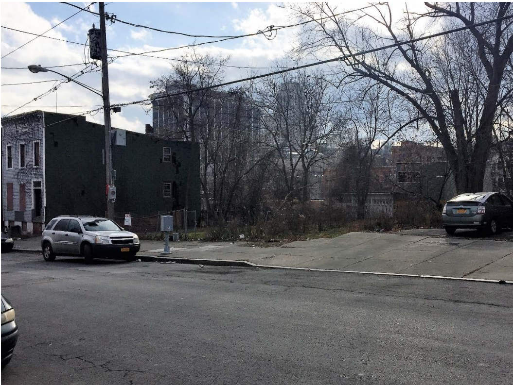
Figure 33. Current Conditions of 288-292 Orange Street The building pictured to the left has since been demolished
